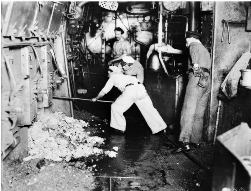
An unidentified stoker scrapes out the ash from the bottom grate in the boiler furnace on HMAS Australia . (Photo c 1918)
